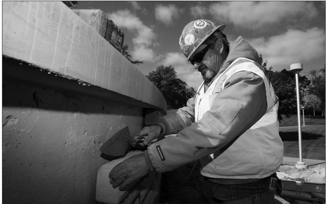
Bob Ansell of Rudolph Libbe set Lannon stone on the Veterans' Plaza, which was dedicated Nov. 11. Located between University Hall and Memorial Field House, the plaza is a place to remember those who have served the nation.
